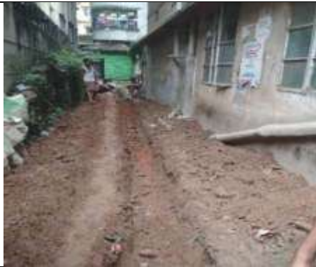
Excavating through open trench method
