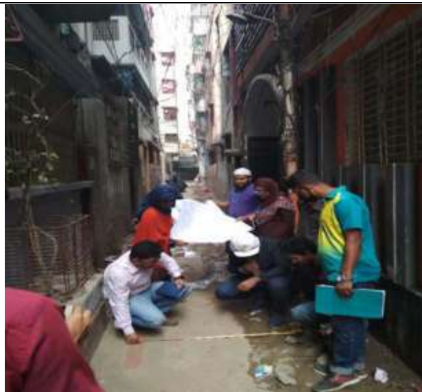
Maintain 1m distance from the AC pipe at DMA 206
