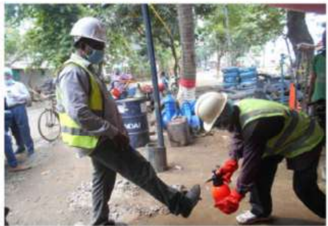
Applying disinfection spray before enter to the site (DMA 206)
