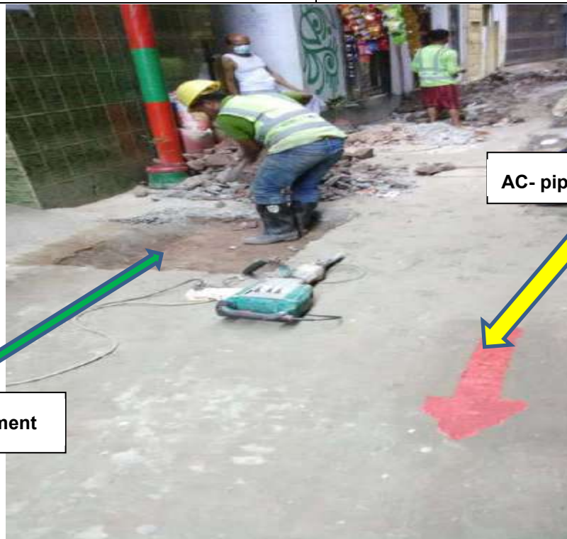
Proper marking of AC Pipes during implementation of DMA 206 under ICB 2.9
