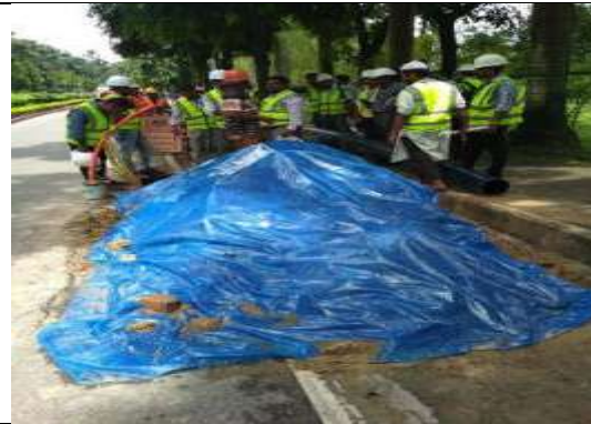
Cover the excavated material
