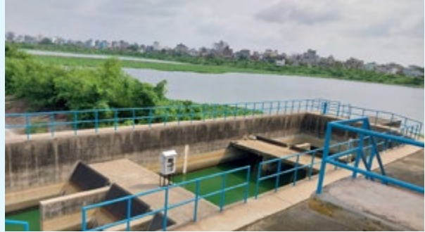
Pagla Sewage Treatment Plant (PSTP)
